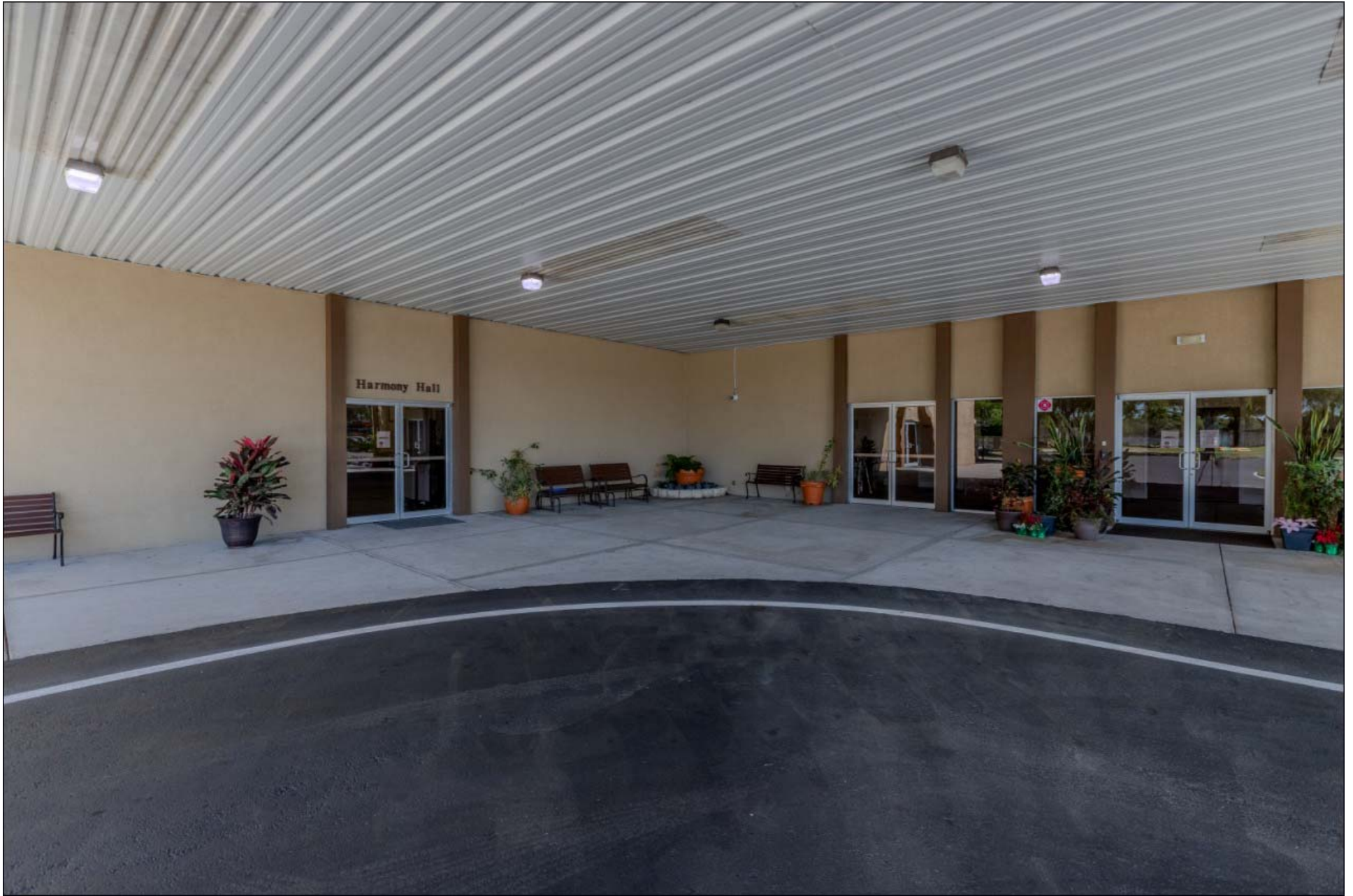
Canopy Drop-off & Pick-up zone
