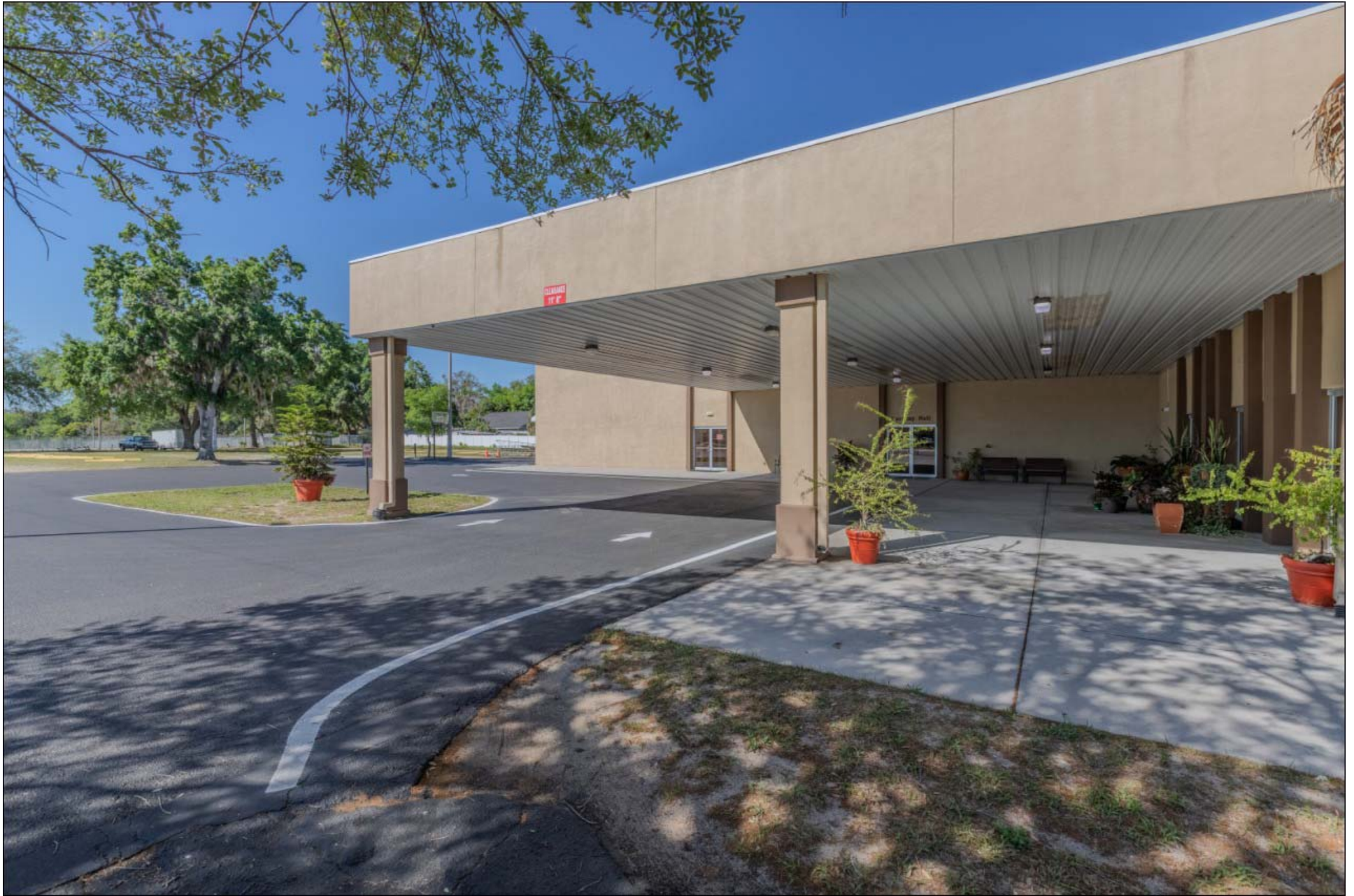
Canopy to the larger Back Parking Lot (the back wall left & right glass doors enter into the Youth & Harmony Halls respectively)
