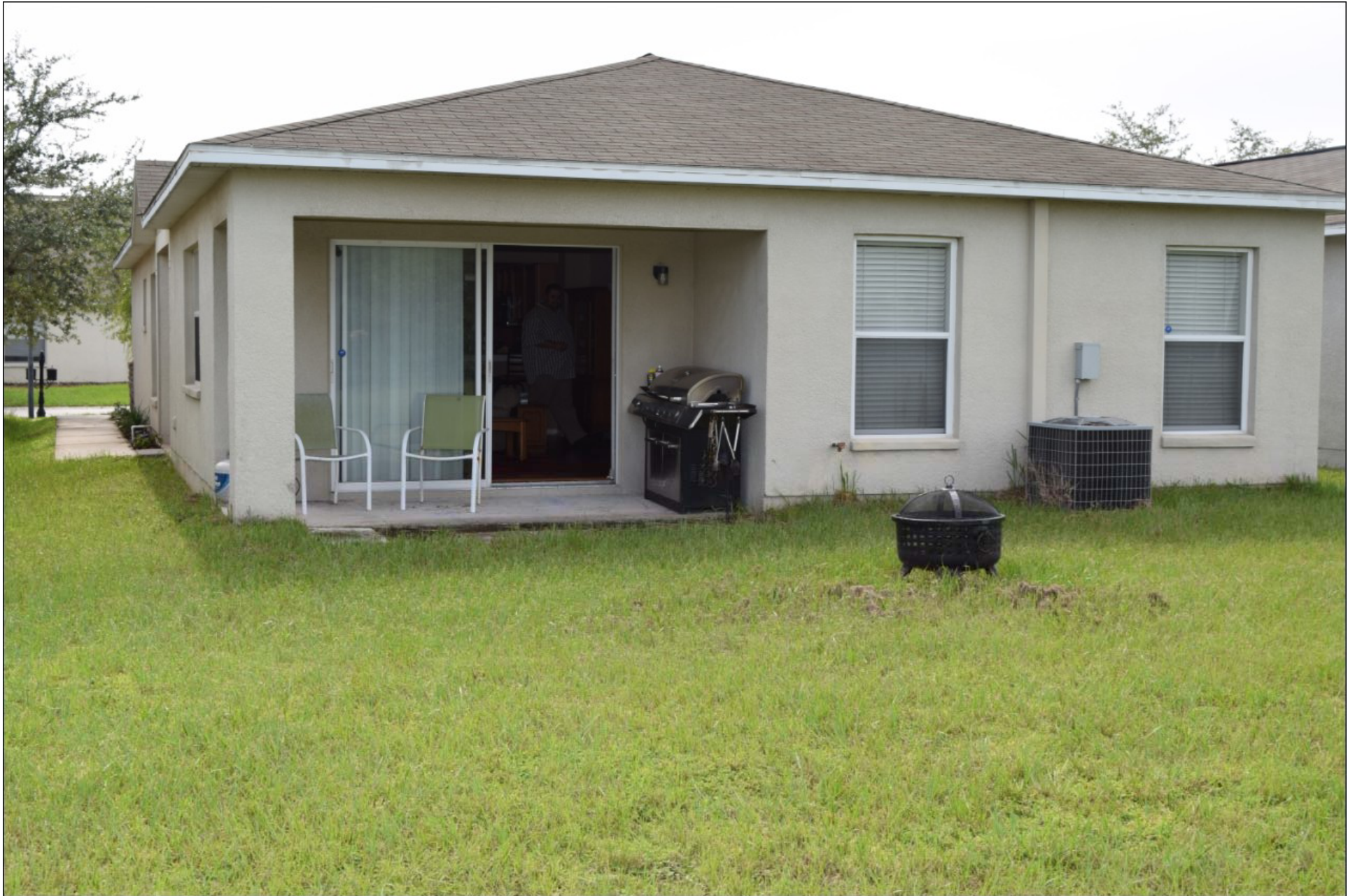
Patio overlooking large back yard & conservation view
