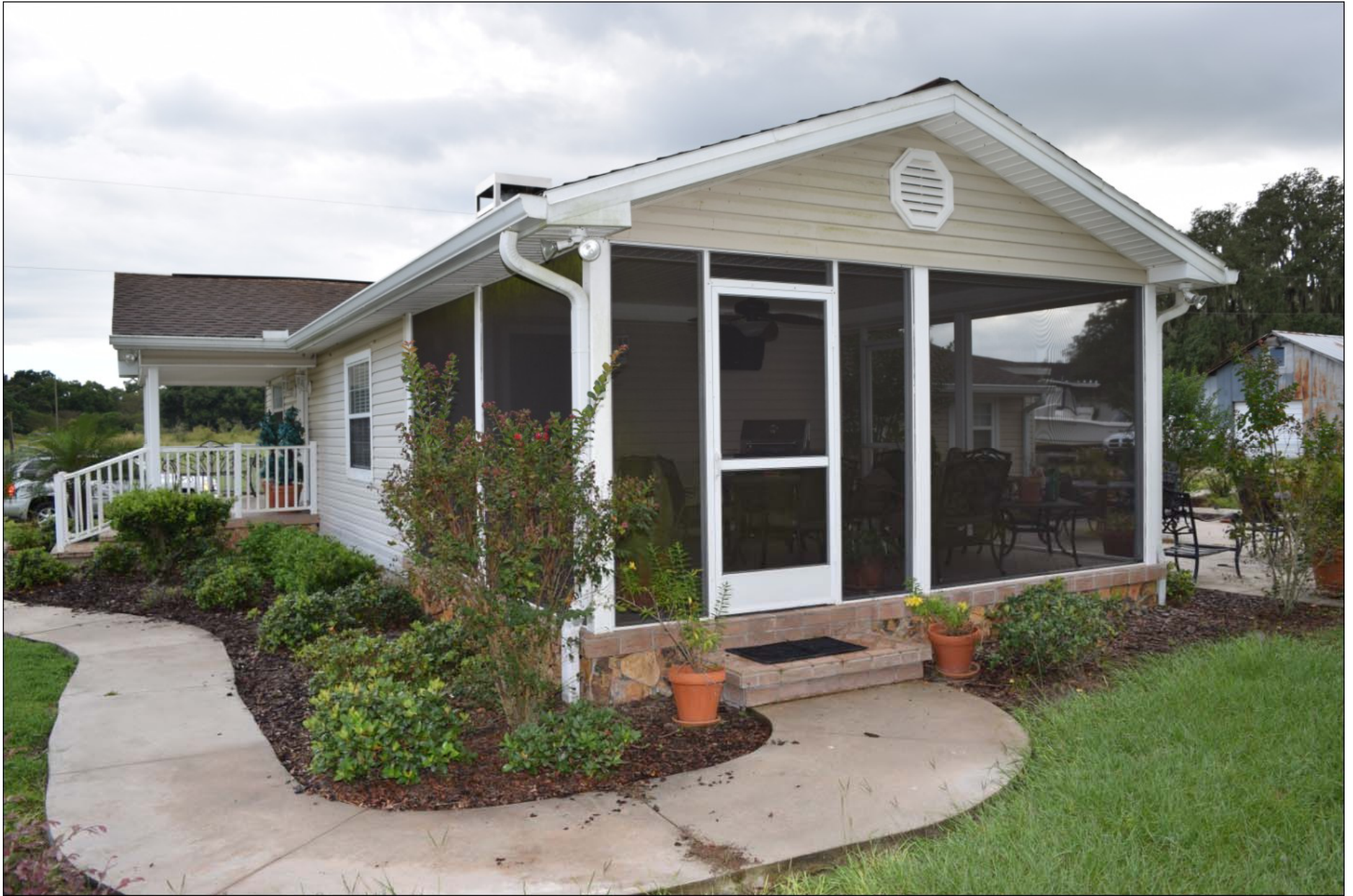
North Side Screened in Patio
