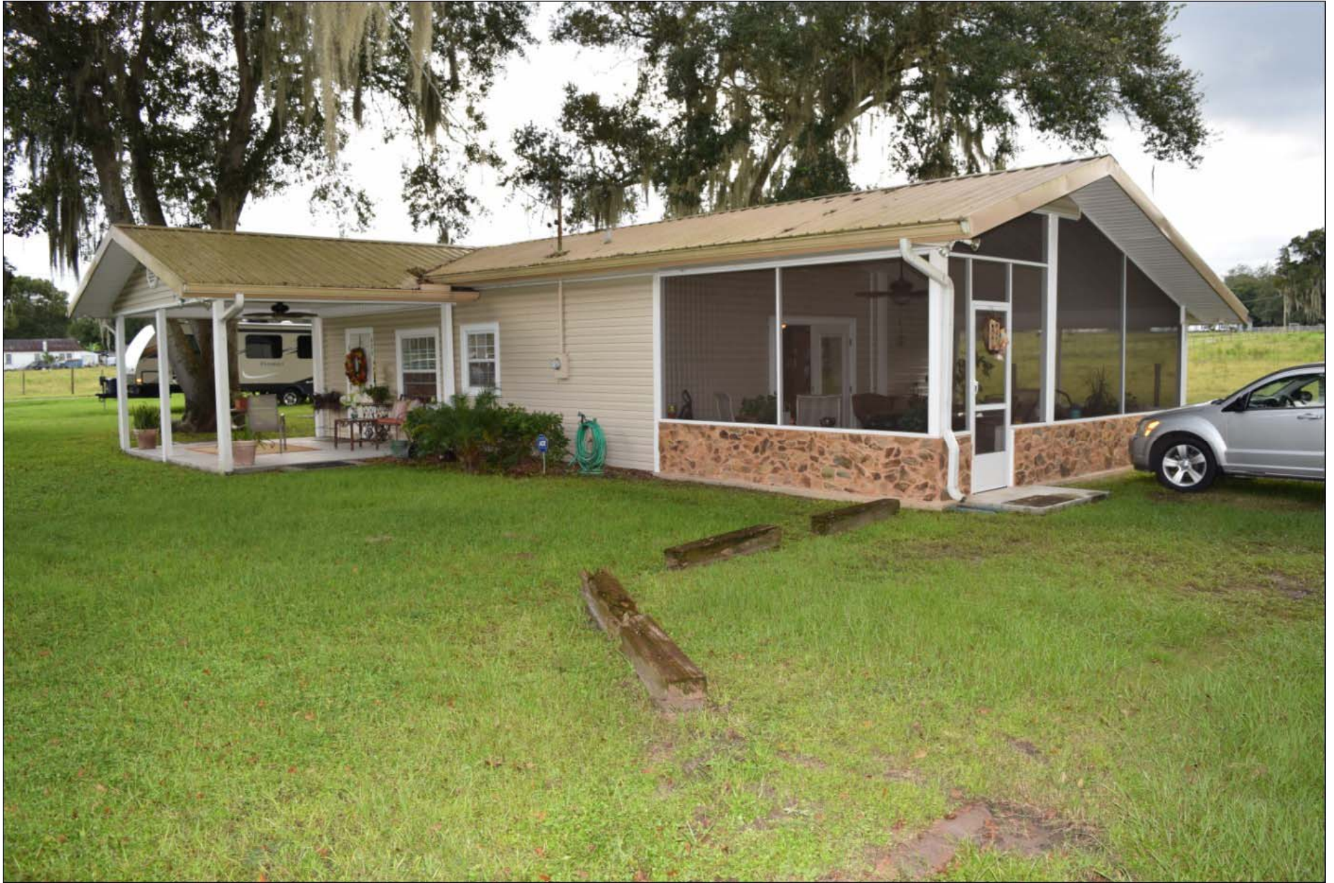
Front / North Side View
