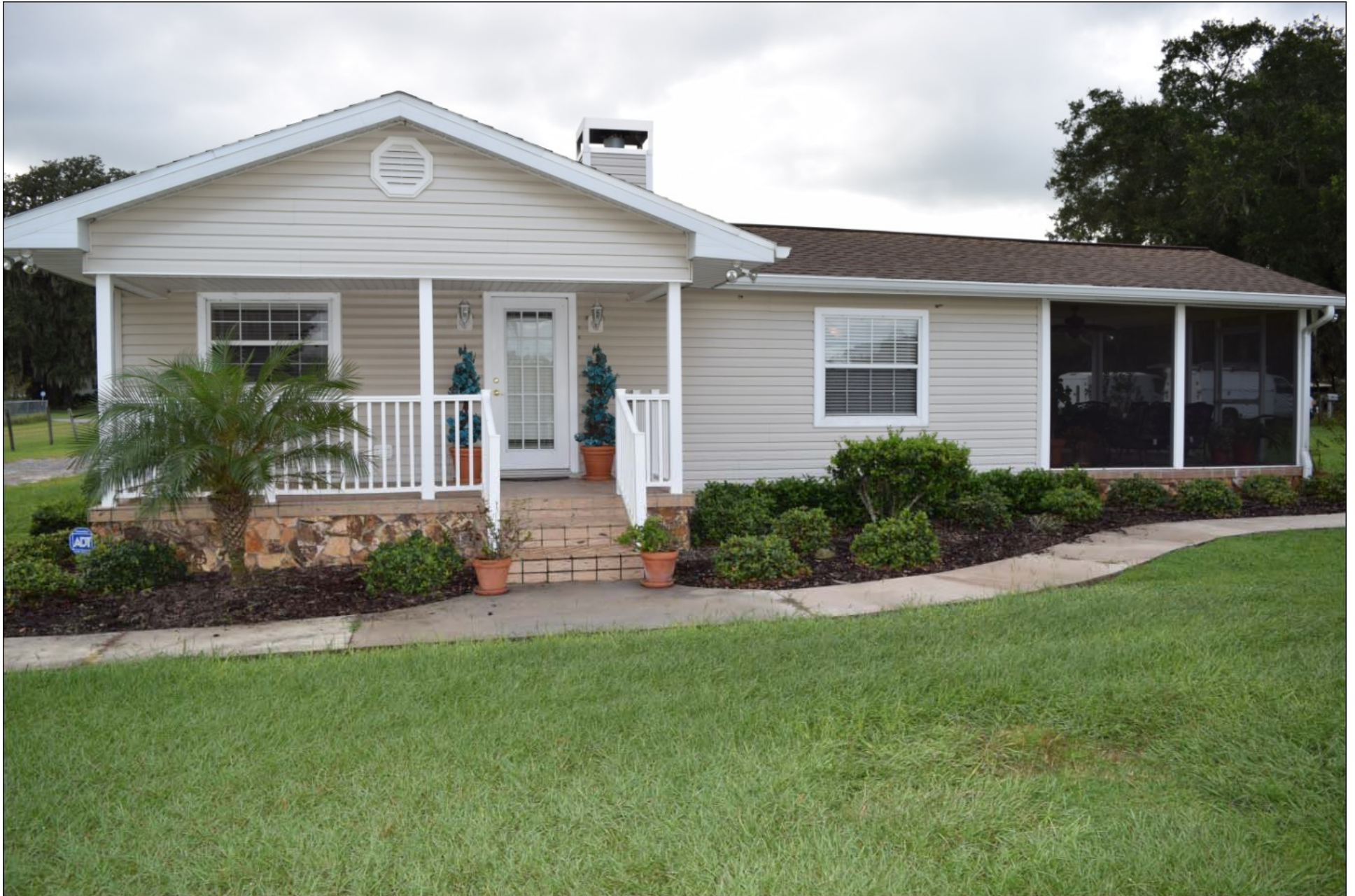
MAIN HOUSE – Front View
