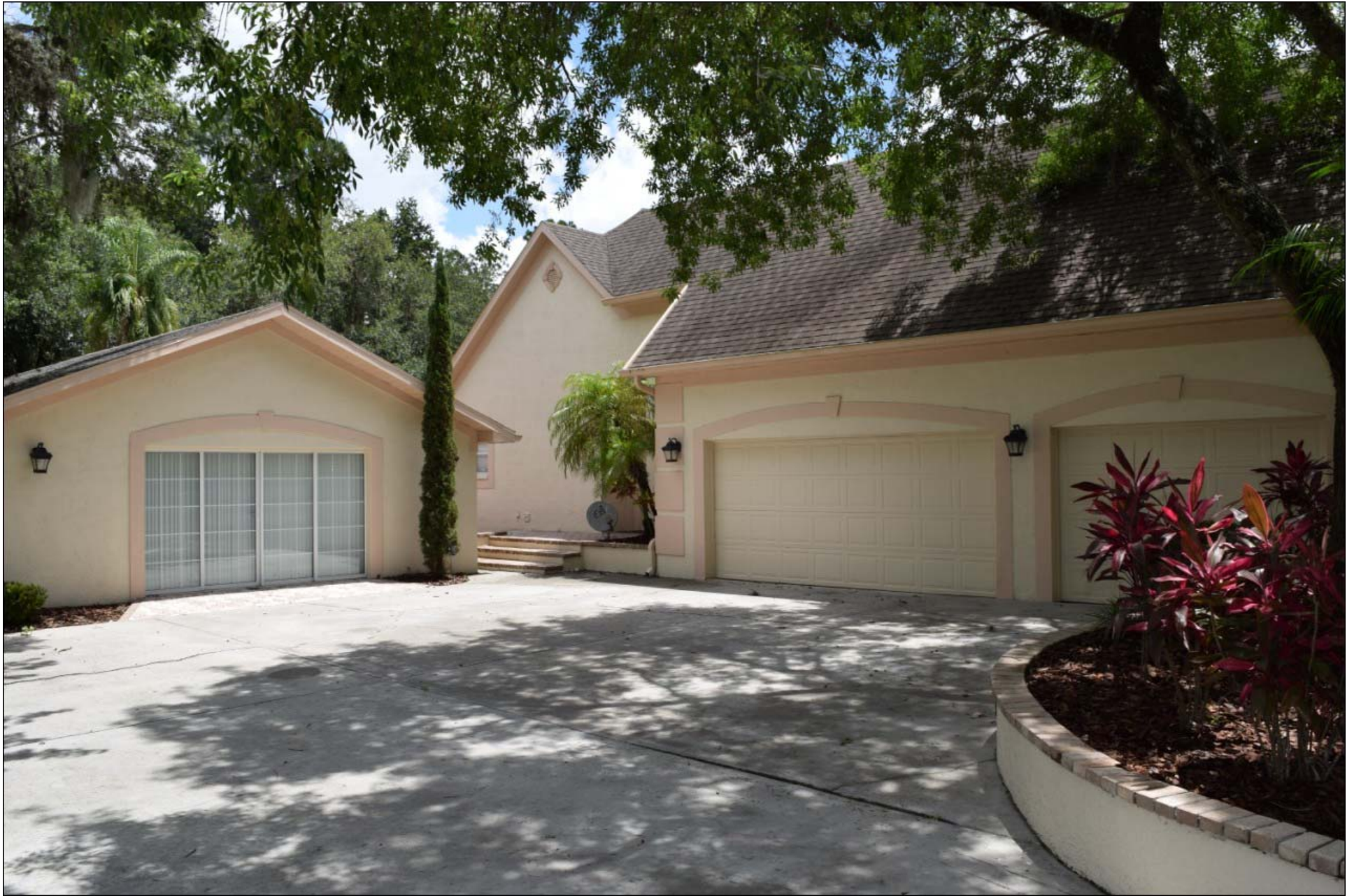
Side 3 Car Garage and Large Bonus Room with Sliding Doors
