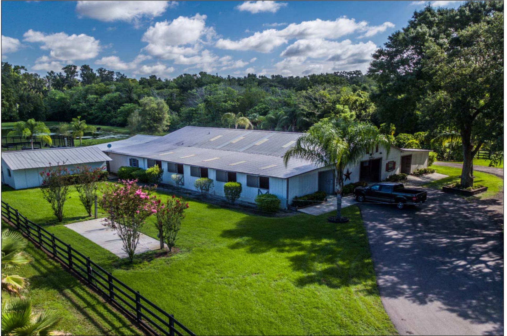
State of the art 21 Stall Barn with ' external stall windows ', Storage Shed & Guest Cottage
