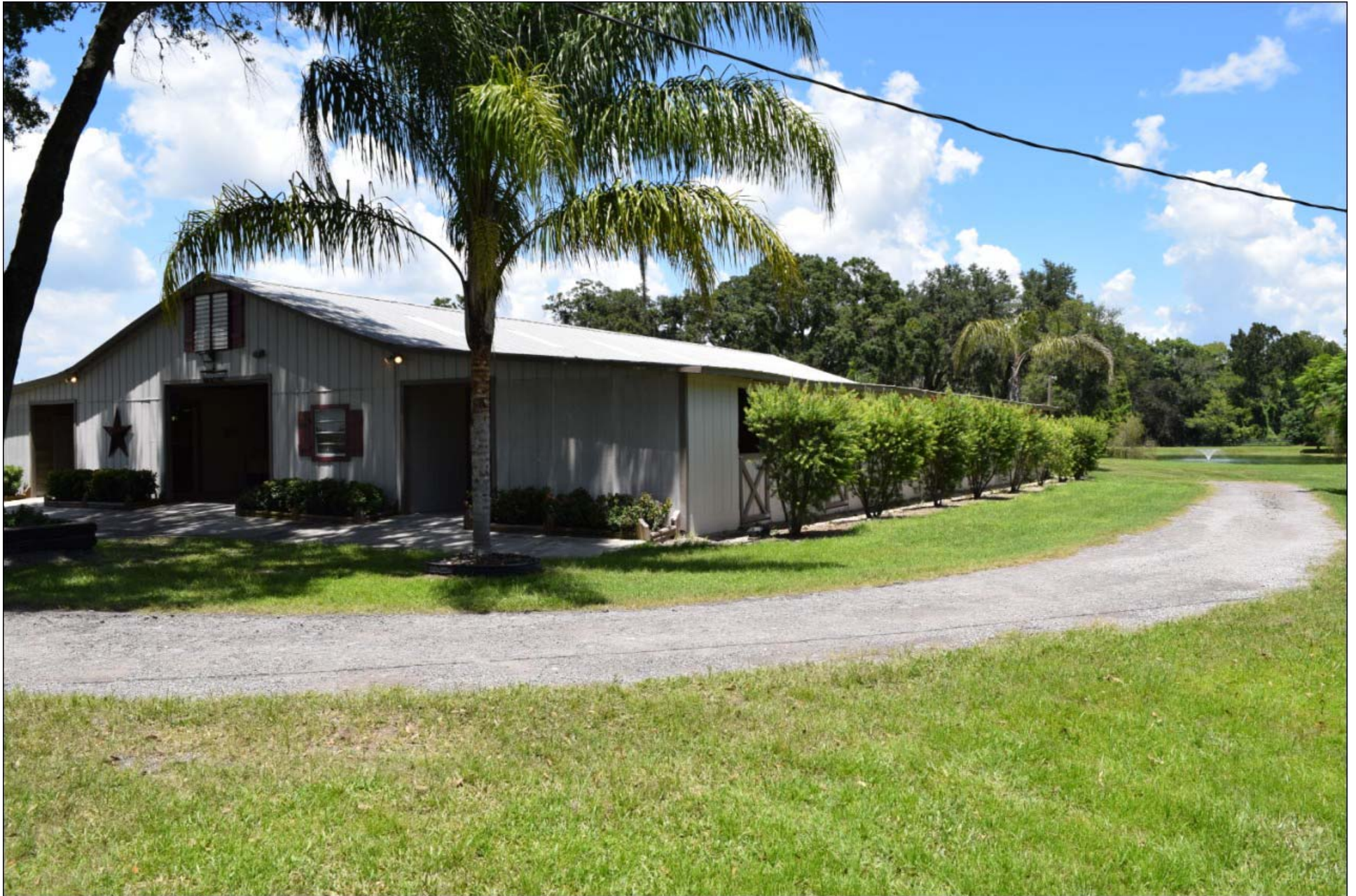
East side of Barn with ' external stall windows '
