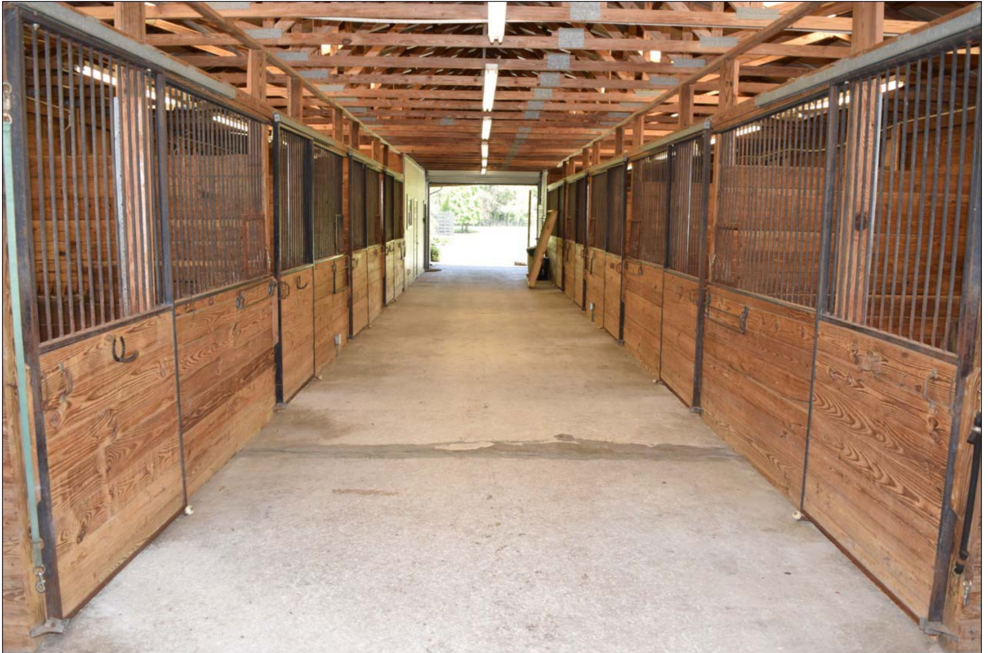
Electronic Entrance Security Gates, 21 Stalls with 'back social & cross ventilation windows' for horses calmness & comfort
